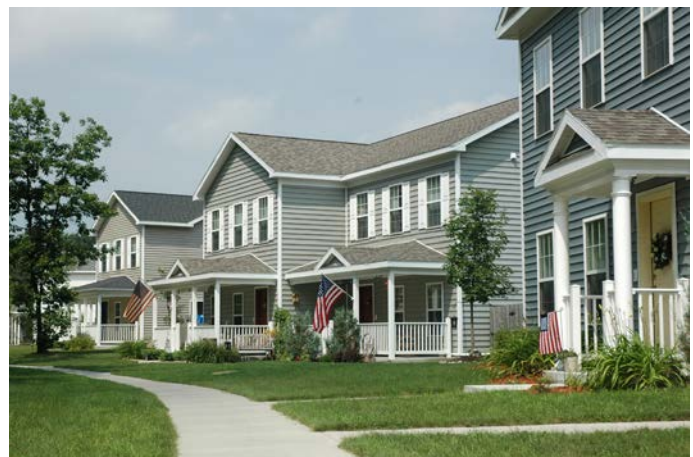
New construction workforce housing
