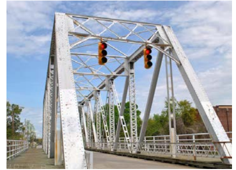
3 North sixth Street Harry Forden Bridge
