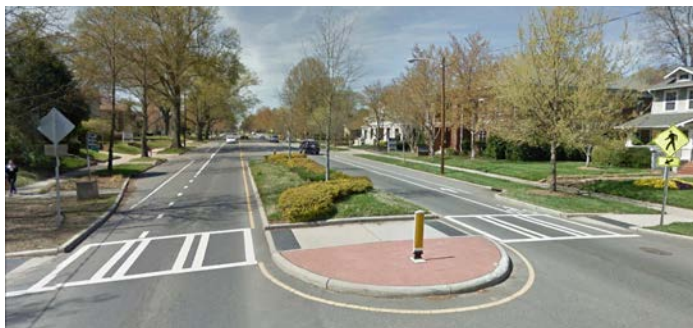
East Boulevard had two of its lanes removed to make traffic flow better and improve pedestrians safety (Charlotte, NC).
