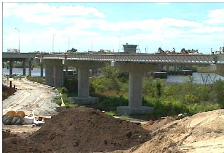
Martin Luther King, Jr. Parkway Construction 2003
