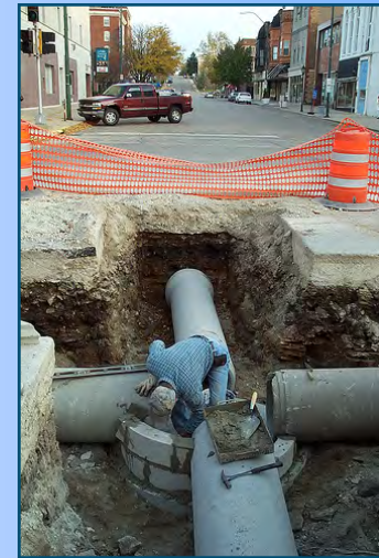
Sanitary sewer construction
