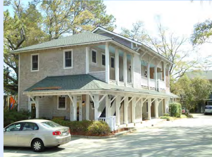
Wrightsville Avenue Office Park: 26 ft Zoning: O&I-1, Office & Institutional-1
