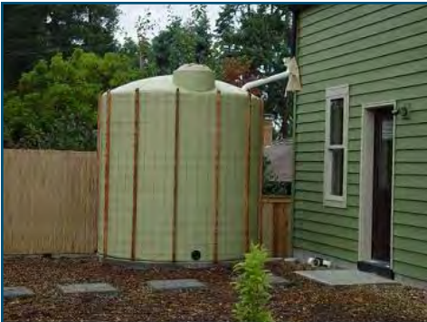
Cistern to collect rainwater for future use
