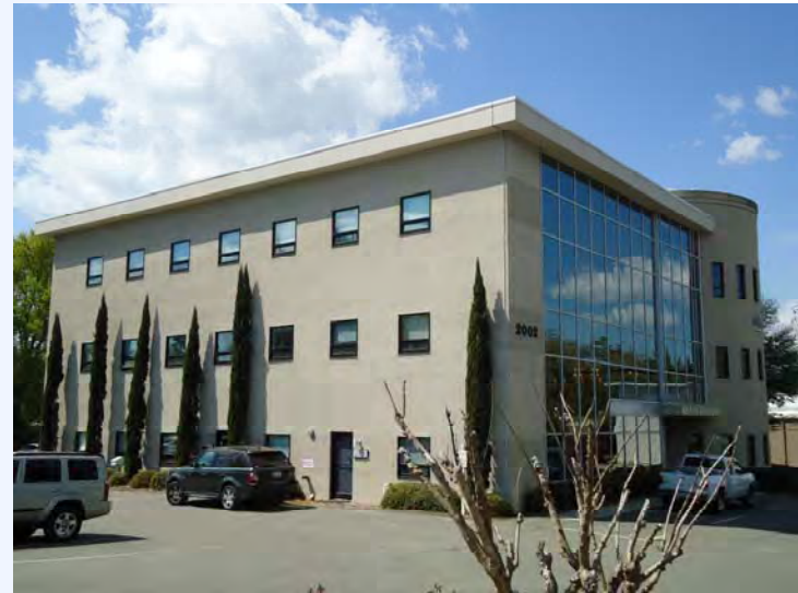
Sea Tower Office Building: 44 ft Zoning: C-5, Commercial (Wrightsville Beach)
