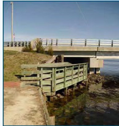
Pedestrian walkway under Corbett Ave (NC 24) in Swansboro, NC
