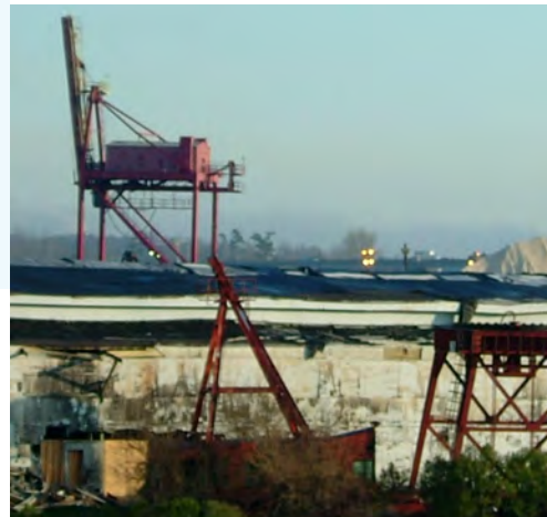
Industrial uses to the north of downtown offer prime opportunities for development.
