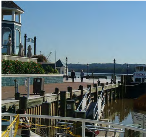
A partnership of public infrastructure and private development improved this waterfront.
