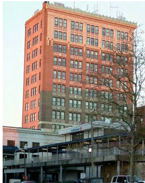
Several buildings designed as 10 or more stories punctuate the Wilmington skyline.
