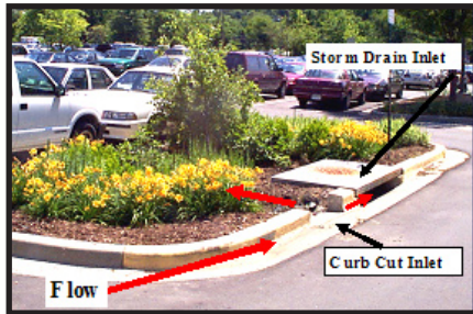
Figure 5-8 Off Line Design – Runoff enters the curb cut. When the cell is full, water bypasses the bioretention area and enters the storm drain. Source, Larry Coffman.
