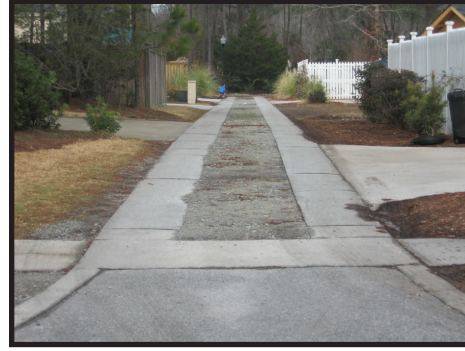
Figure 4-15 Ribbon driveway in Demarest Village in Wilmington, N.C.
