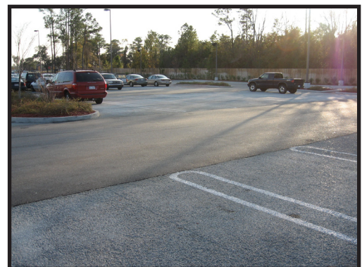
Figure 5-20 Porous concrete in parking stalls at Costco in Wilmington. .
