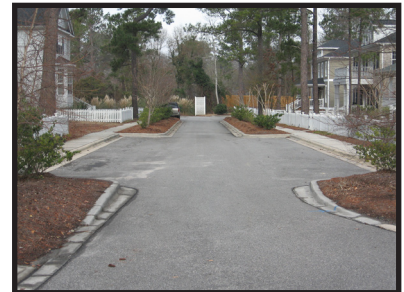
Figure 4-7: Bioretention cells used for stormwater runoff and traffic calming in Demarest Landing in Wilmington, NC.
