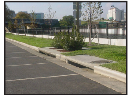
Figure 5-10 Proprietary bioretention system. Source Americast, Filterra.
