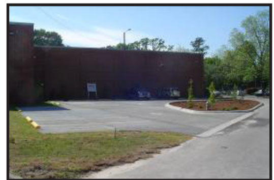
Figure 3-9 Completed porous parking and bioretention area at YMCA. Source NCSU.
