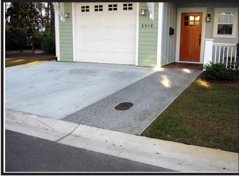
Figure 4-14 Porous Pavers in driveway at Preservation Park in Wilmington, N.C.
