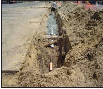
Figure 3-6 Underdrain installation at Port City Java. Source NCSU.
