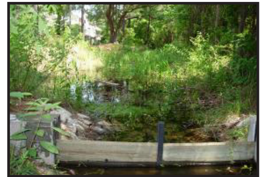
Figure 3-18. Stonestrow constructed wetland after completion. Source NCSU.
