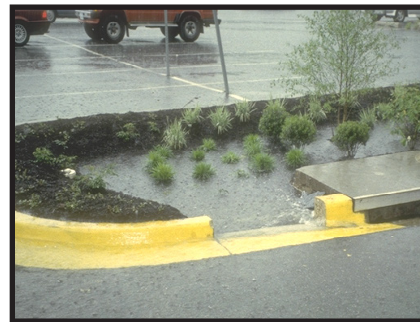
Figure 3-4. Completed bioretention cell with plantings. Source Larry Coffman.
