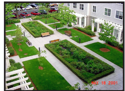
Figure 3-23 Center landscape feature is a bioretention cell with detention. Source Portland, OR BES.
