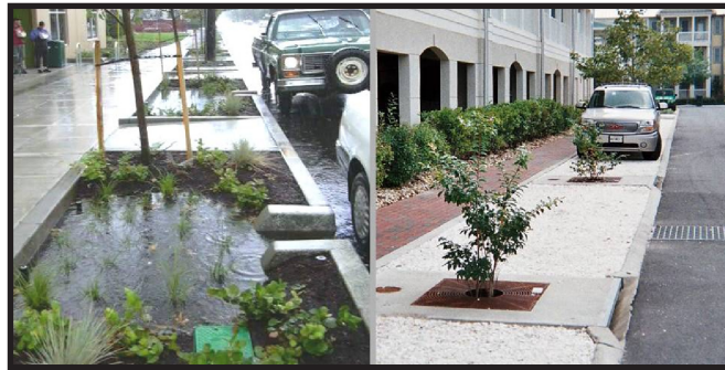
Figure 4-6 Bioretention planter boxes. Sources City of Portland, OR BES and Ocean City, MD Filterra™
