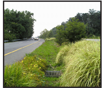
Figure 5-11 Vegetated swale in a roadway median. Source LID Center
