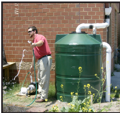
Figure 3-13. Installation of cistern at Gregory Elementary School
