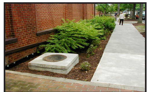
Figure 5-4 This bioretention cell intercepts downspout and walkway runoff. Note the overflow. Source LID Center.
