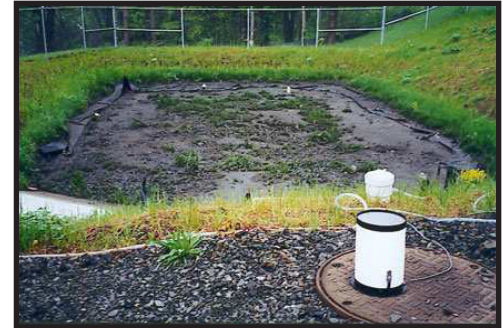
Figure 5-31: Sand filter installation
