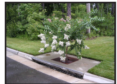
Figure 4-11 Bioretention system in a concrete box and used as an infiltration system. Source Americas Filterra.
