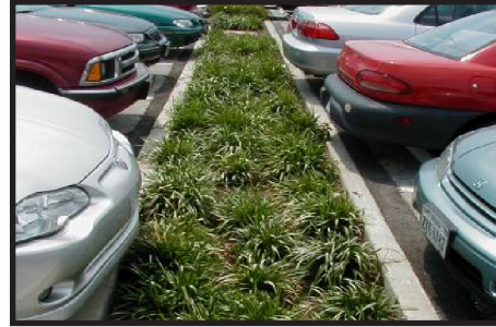
Figure 3-22. Completed bioretention cell at Navy Yard. Bioretention cell used for filtration only. Source LID Center.
