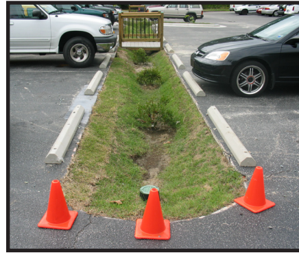
Figure 3-7 Completed Port City Java bioretention cells with plantings. Source NCSU.
