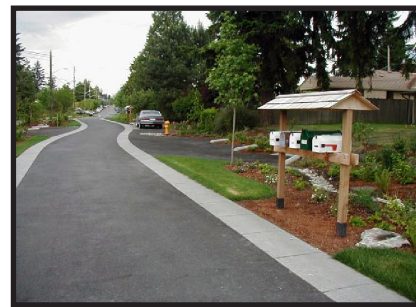
Figure 3-28 Completed Seattle retrofit streetscape. Source Larry Coffman.
