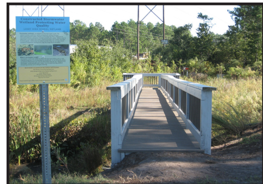
Figure 3-16. Laney constructed wetland after completion. Source New Hanover County Planning.
