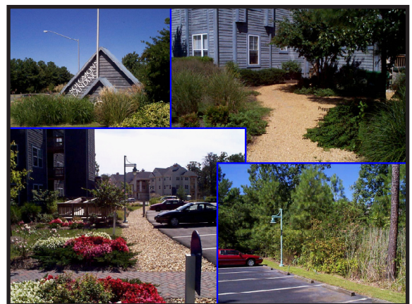
Figure 2-12 This high-density residential community in the Chesapeake Bay watershed is a zero-discharge design that was constructed for sandy soils and a high ground water table. The design included infiltration devices under the buildings, parking lots, and side-walks; conservation and buffers areas to treat runoff; rain gardens and porous pavements.
