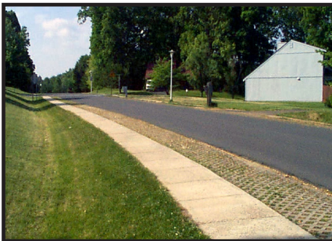
Figure 4-16 Narrow road section with a shallow swale, sidewalk, and porous paver shoulder.
