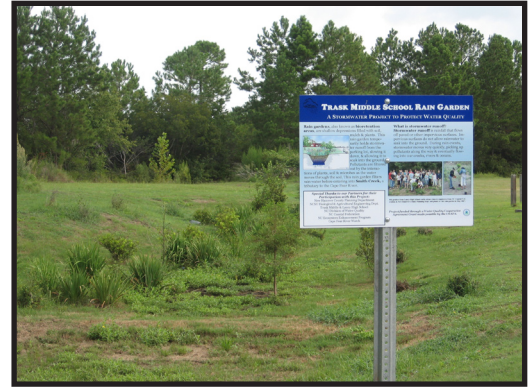
Figure 3-14. Completed Trask bioretention area. Source New Hanover County Planning.
