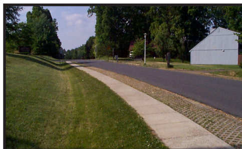
Figure 4-5 Narrow road section with a shallow swale, sidewalk, and porous paver shoulder.
