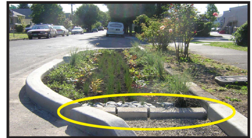
Figure 4-9 Example of a bioretention cell within the road right-of-way. Source Portland, OR.
