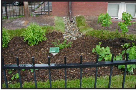
Figure 3-21 Disconnected gutter and bioretention area at Navy Yard. Source LID Center.
