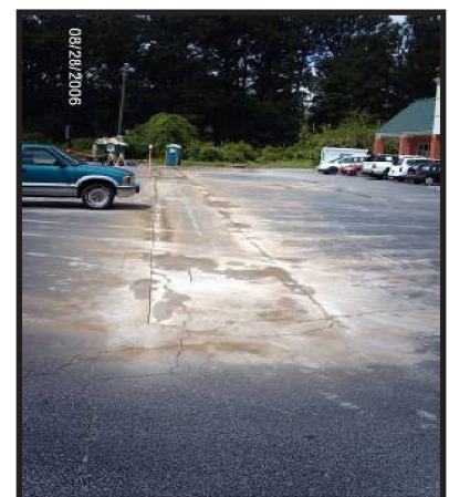
Figure 3-5. Port City Java parking lot prior to retrofit. Source NCSU.
