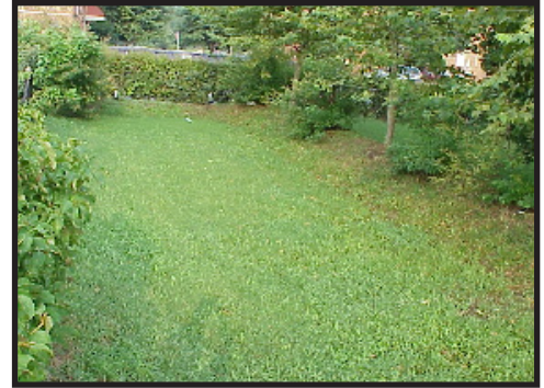
Figure 5-5 Grass-lined bioretention cell. This cell has greater storage depths of 2.5 feet for additional storage. Source Larry Coffman.
