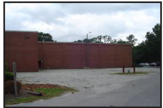
Figure 3-8 YMCA overflow parking area prior to retrofit. Source NCSU.
