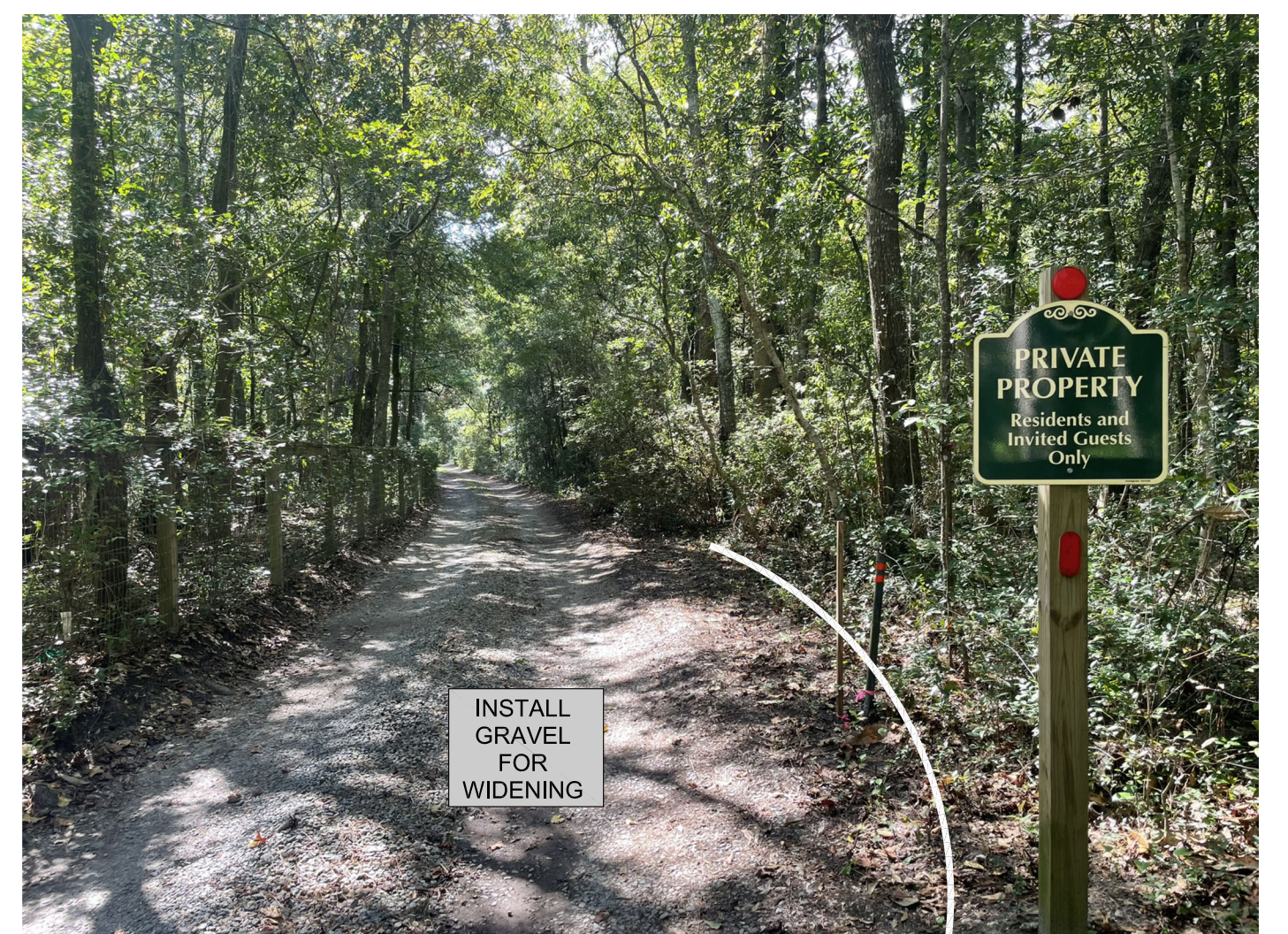
Station 1+85± Private Access Drive
