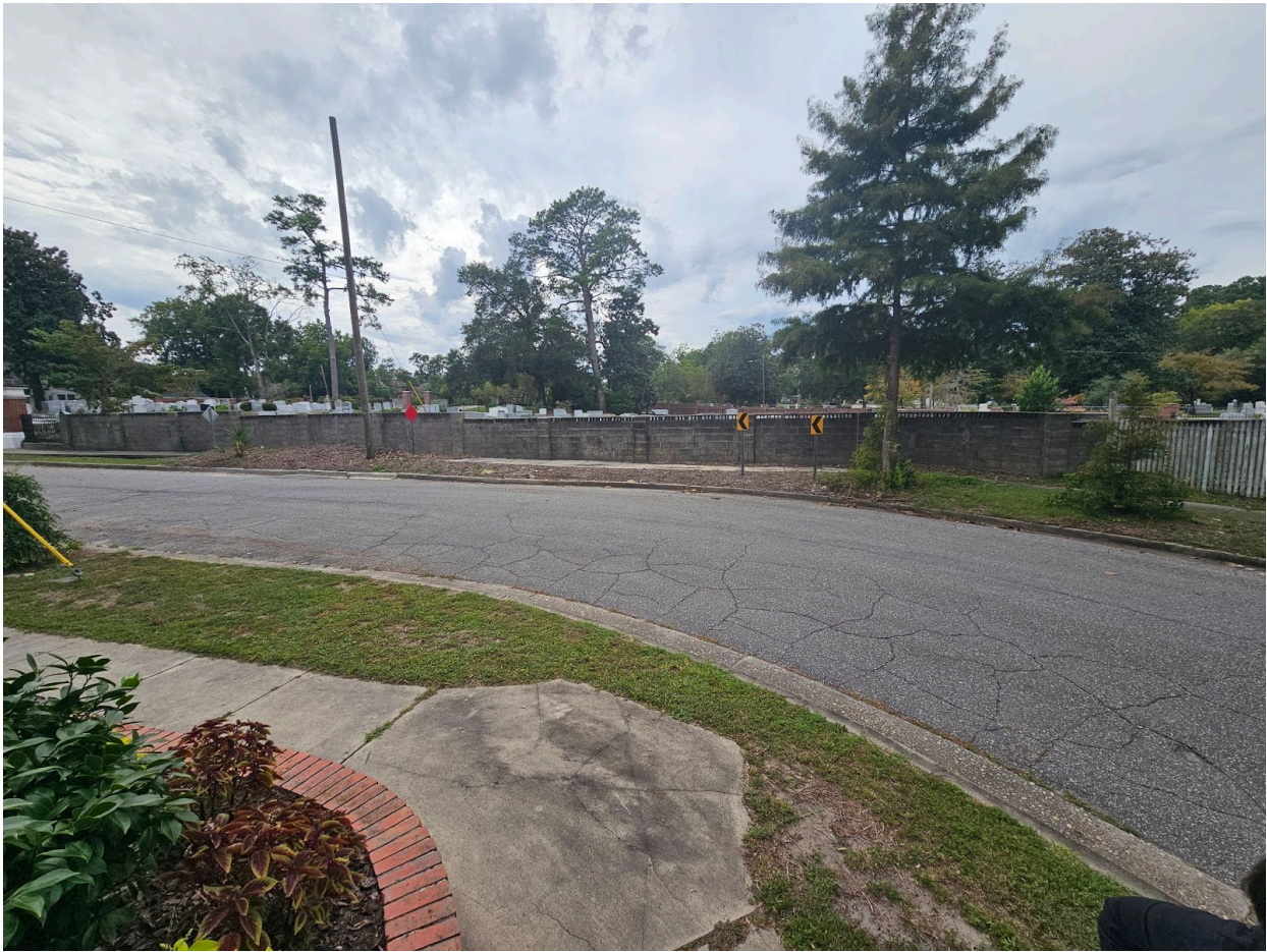
Picture 1 - Existing cinder block wall
