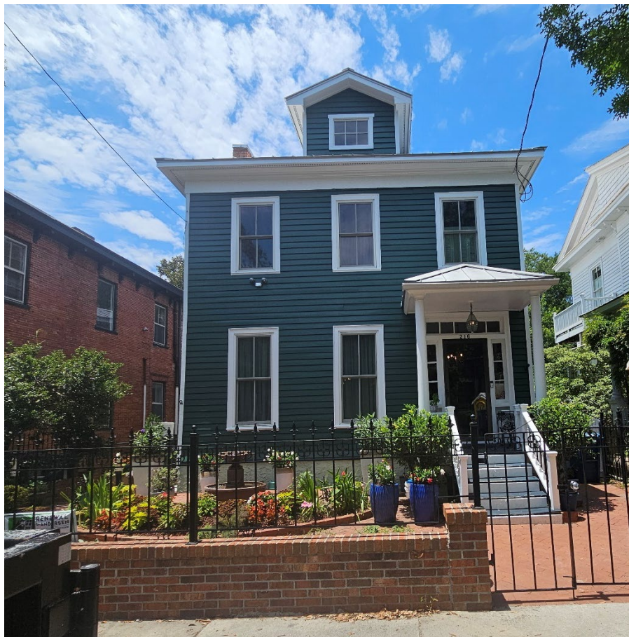
216 South 3 rd Street, Front (east) Façade, June/2024
