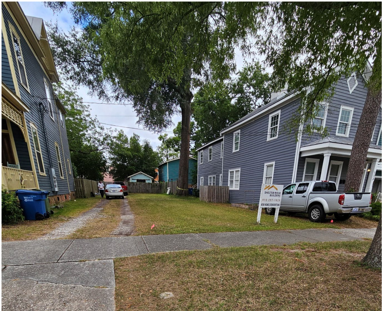
111 North 7 th Street, Front (east) Façade, June/2024
