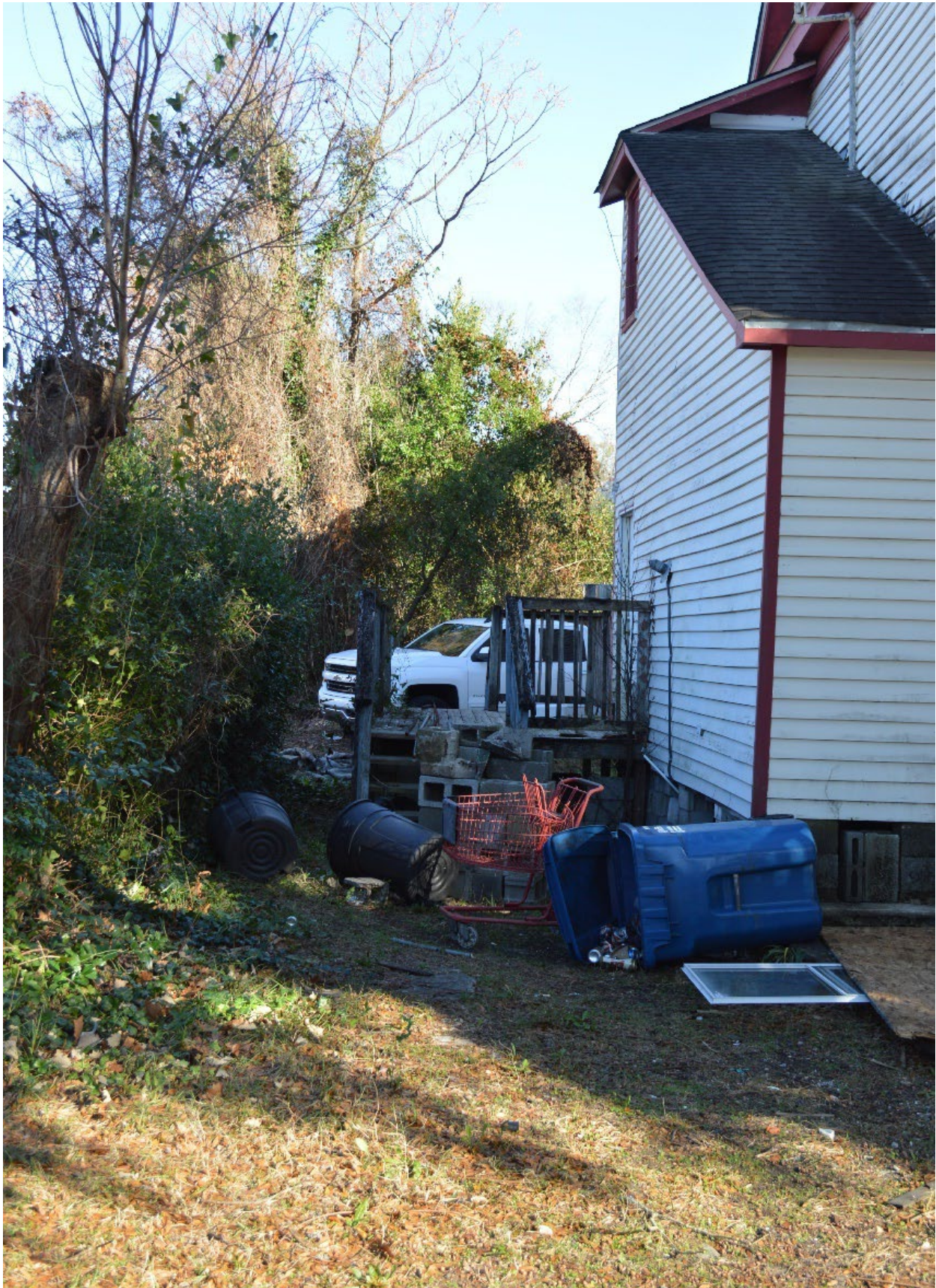
416 North 5 th Avenue, Side (north) Yard, City Records, 2022
