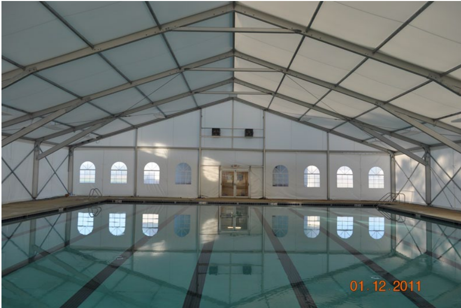
Image 1. Sample photo custom aluminum fabric clad pool cover
