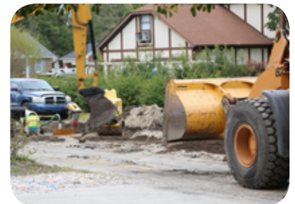
Drainage work in Pine Valley neighborhood
