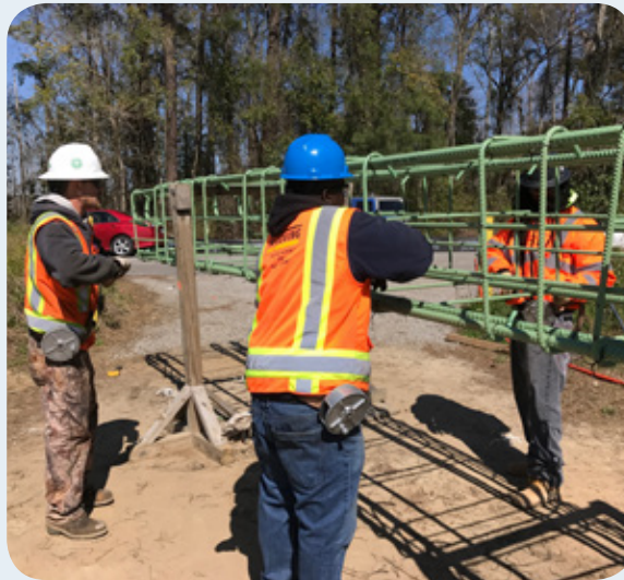
Love Grove bridge project.
