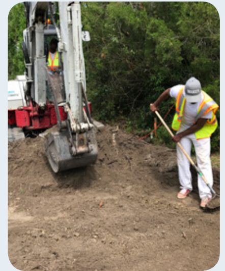
Fairlawn sidewalk project.
