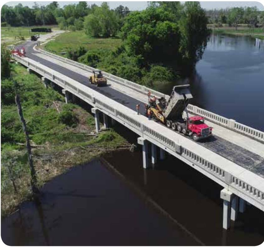
Love Grove Memorial Bridge
