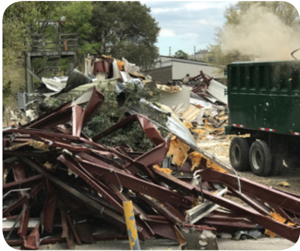
Metal being set aside for recycling during demolition of downtown warehouse
