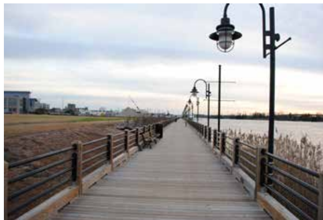
Site photos of the park land and the Riverwalk.
