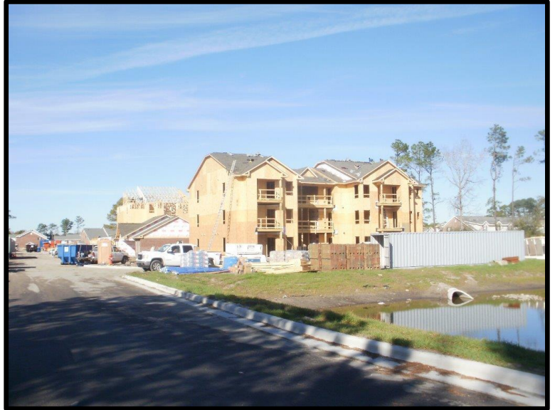
Lockwood Village Under Construction 2015
