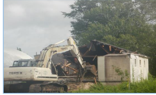
10th & Fanning demolition
