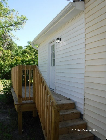
After- Lead-based Paint Remediation/Healthy Homes
