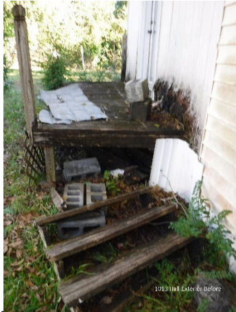
Before - Lead-based Paint Remediation/Healthy Homes
