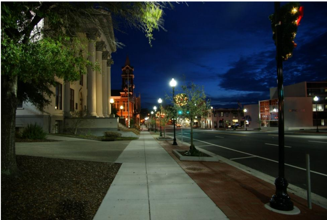
North Third Street Improvement Project featuring LED street lighting Photo Source: Dylan Lee
