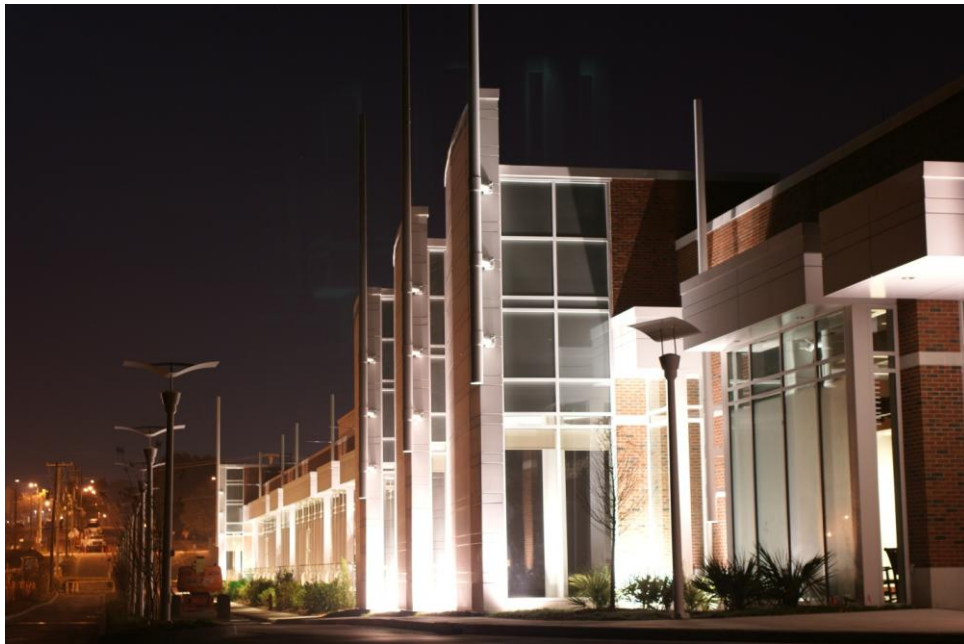
The City of Wilmington's LEED Silver Convention Center Photo Source: Dylan Lee
