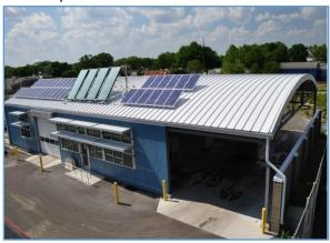
All of the systems are tied into the grid and setup under a net metering rate, meaning when the system is producing energy, any energy that is not utilized on-site is fed back into the grid. In FY17 the systems produced nearly 150,000 kilowatts hours (kWh) of electricity...that's equivalent to offsetting the GHG emissions from 11.1 homes for one year!
