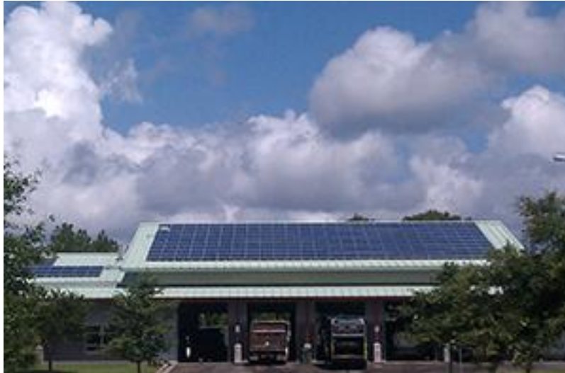
Image 8: City of Wilmington, NC Fleet Management 74 kw solar array
