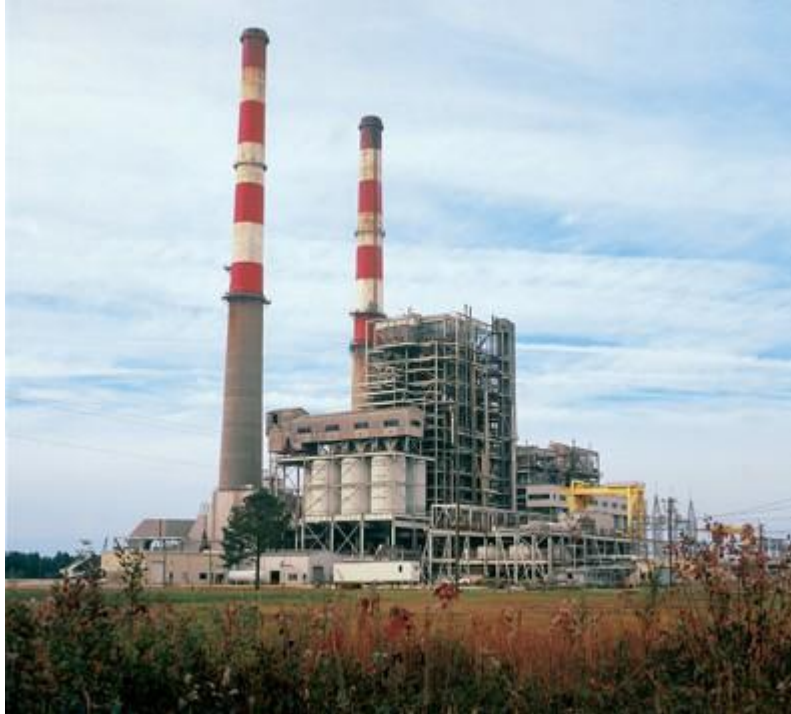
Image 7: Duke Energy LV Sutton outside of Wilmington, NC
