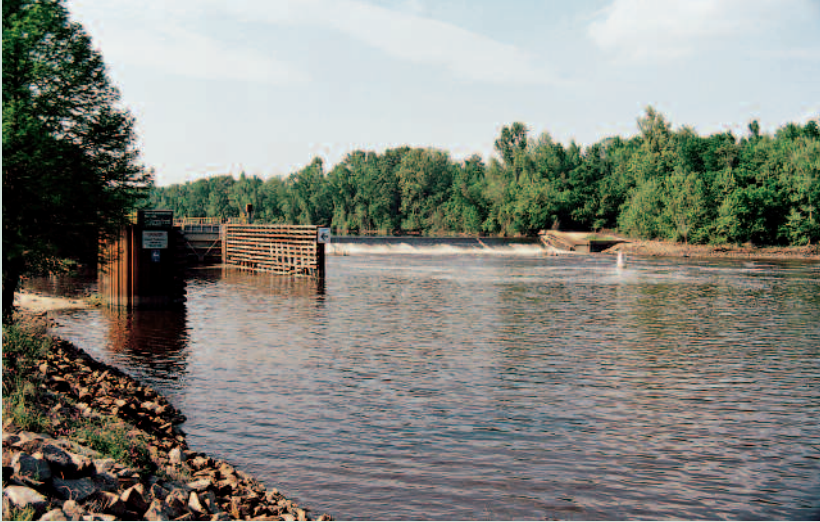
A lock-and-dam on the Cape Fear River near Elizabethtown
