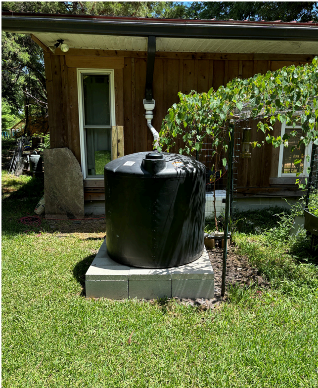
The HOW Program contracts with New Hanover Soil and Water Conservation District to install nature-based stormwater solutions, such as these cisterns and rain gardens that were installed in FY24.
