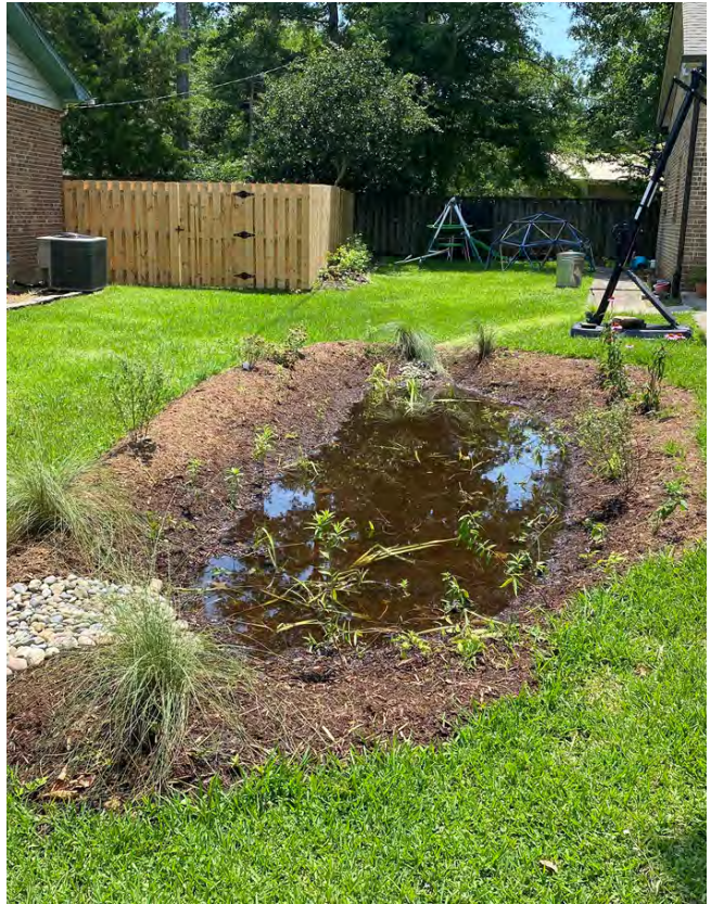
The HOW Program contracts with New Hanover Soil and Water Conservation District to install Stormwater Solutions, such as these cisterns and rain gardens that were installed in FY23.
