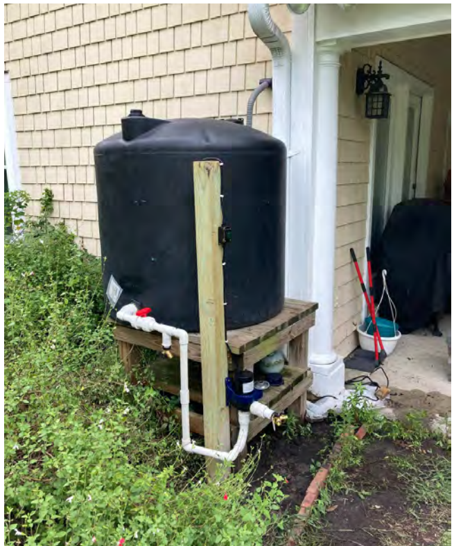
The HOW Program contracts with New Hanover Soil and Water Conservation District to install Stormwater Solutions, such as these cisterns and rain gardens that were installed in FY23.
