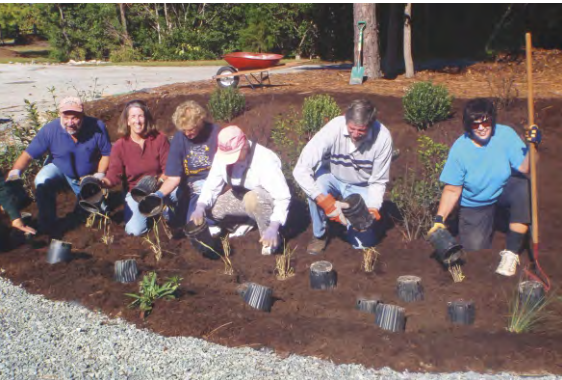
Rain Garden planting at Winding River, Brunswick County
