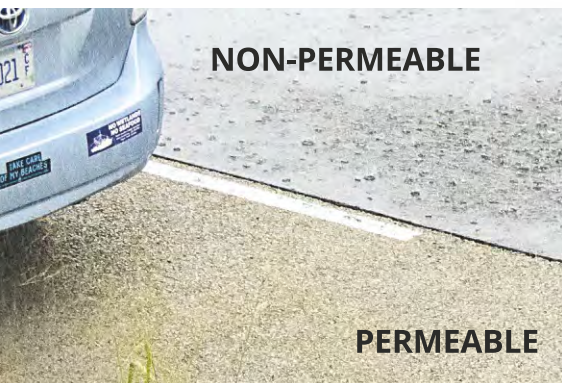
Notice how rainfall soaks into permeable pavement
