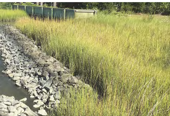
Pine Knoll Shores residential shoreline after restoration
