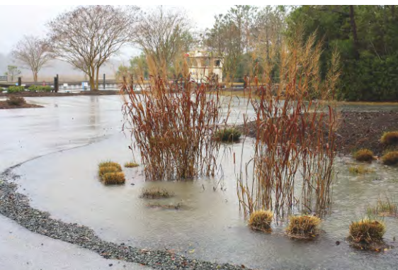
Rain Garden during 1.5" rain
