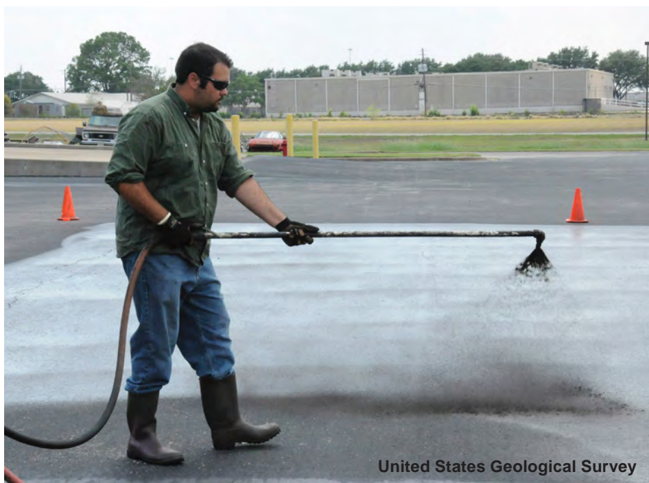
Figure 3. Sealant is applied to a parking lot.
