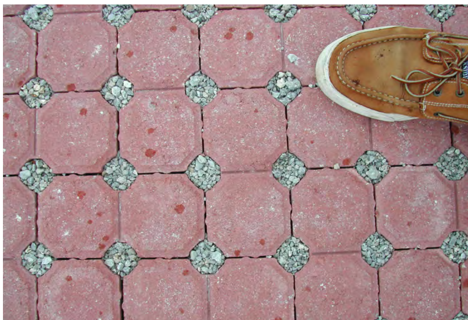
Figure 6. A parking lot with interlocking pavers in Swansboro, N.C.
