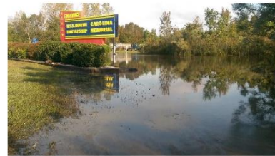
Flooding in Wilmington, NC
