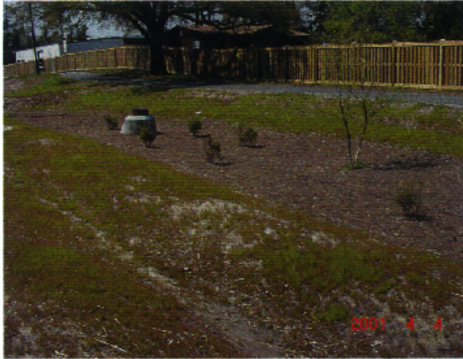
Fig. 5-1. Park Avenue Project bioretention area
