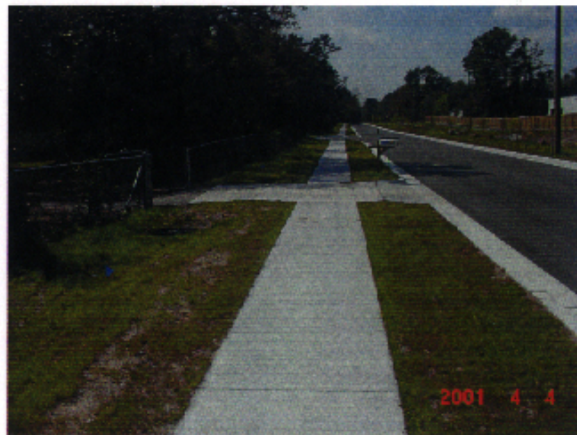
Fig. 13-1. Typical Sidewalk Requirement
