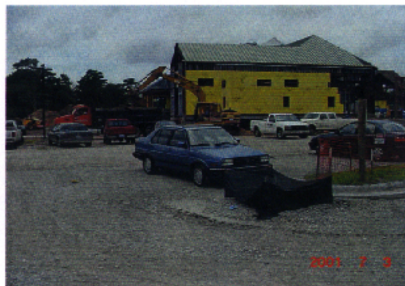
Fig. 19-1. Erosion control measures at construction site
