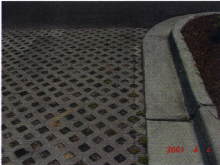
Fig. 6-3. Examples of Turf stone pervious parking material
