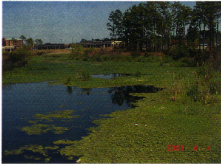
Fig. 11-1. Open space: a regional storm water facility at Silver Stream
