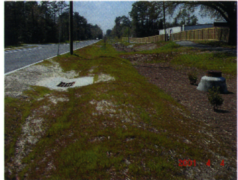
Fig. 5-2. Park Avenue Project grass swale
