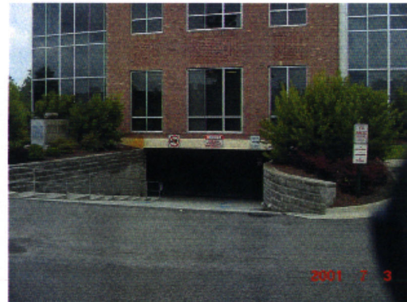
Fig. 9-1. Shipyard Commons office building with parking underneath
