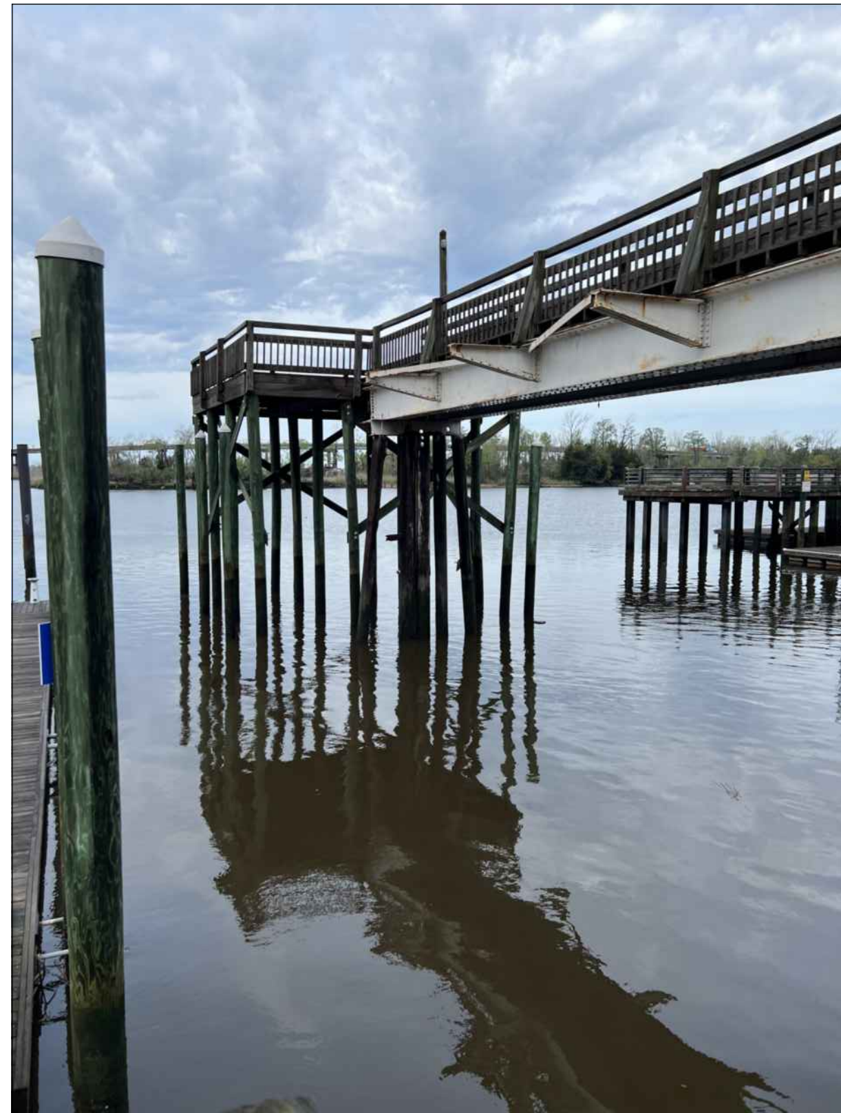
1 SOUTH SIDE OF PIER C201
